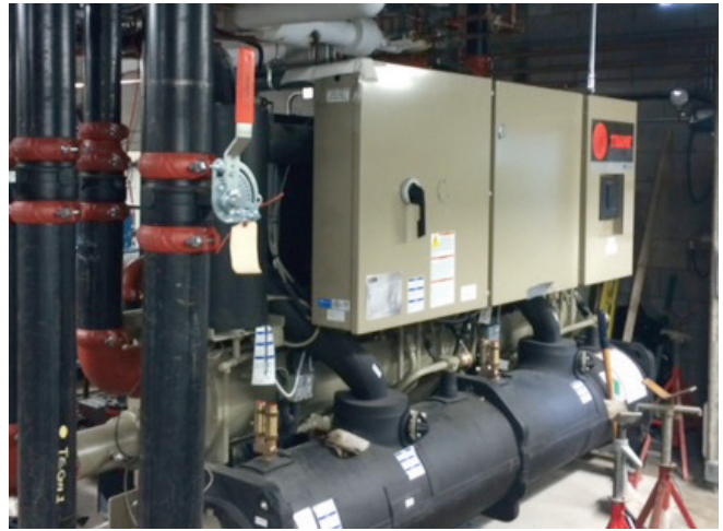
A Trane Series R Helical Rotary Water-Cooled Chiller, used for the centre's geothermal application, is able to maintain tight tolerances for precise temperature control and is also well suited for heat recovery.
