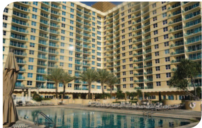
The Wave Condominium sought to upgrade its aging systems to reduce energy costs and increase comfort for residents.
